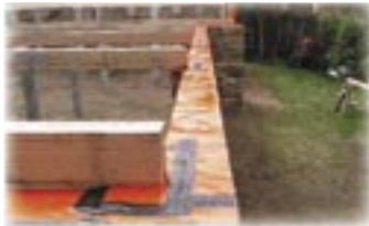
bearers and joists
