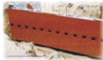
retaining wall installation
