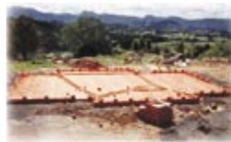
Kordon TMB - full under slab
