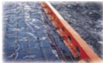
Kordon TB - in-fill slab
